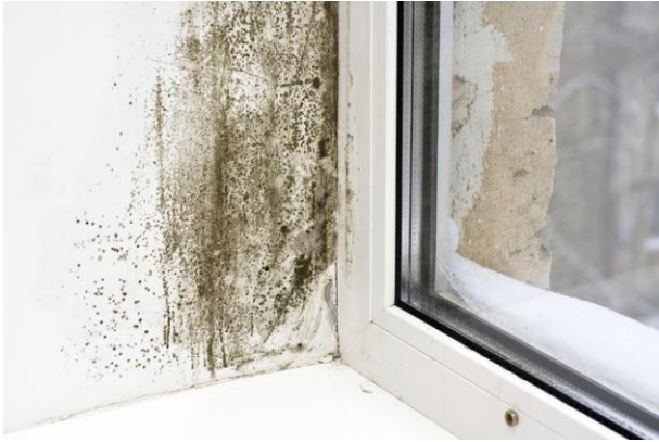
Mould on Reveal (fig1.0)
